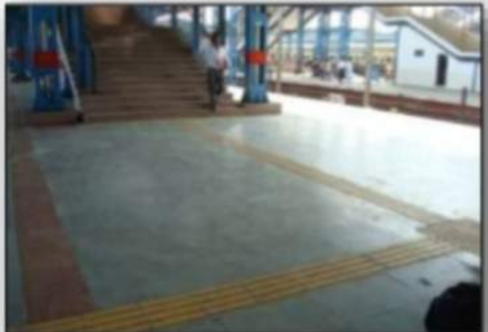
Placement of tactile warning and guiding blocks
