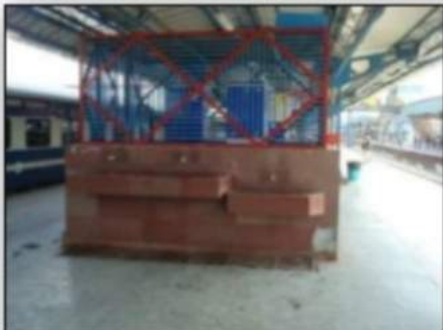
Drinking Water counters at two levels
