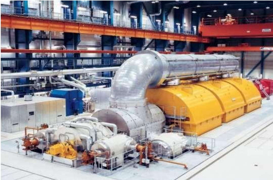
Figure 82: Turbogenerator
