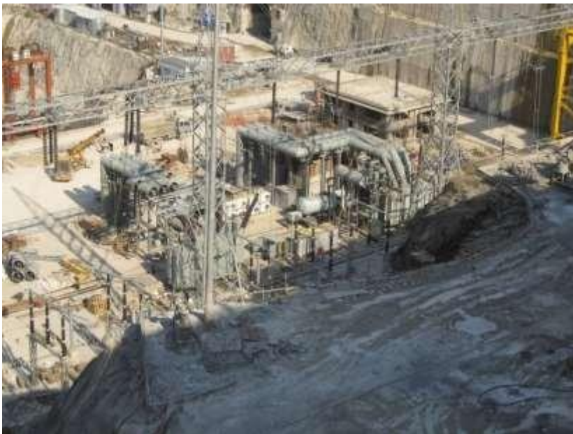
Figure 13: A switchyard under construction
