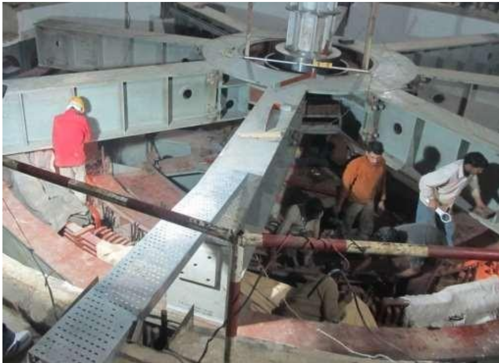
Figure 80: Hydrogenerator under construction
