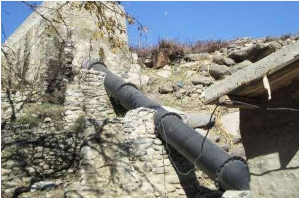
Figure 6: Forebay with Penstock
