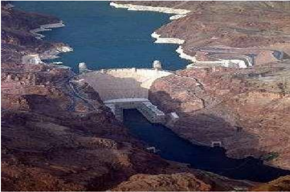
Figure 3: Arc Gravity Dam
