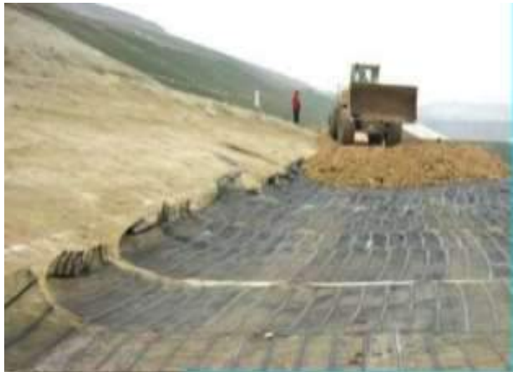
Use of grogrid for soil reinforcement
