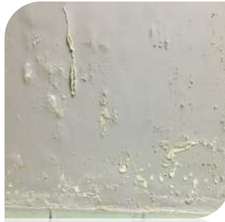
Efflorescence
