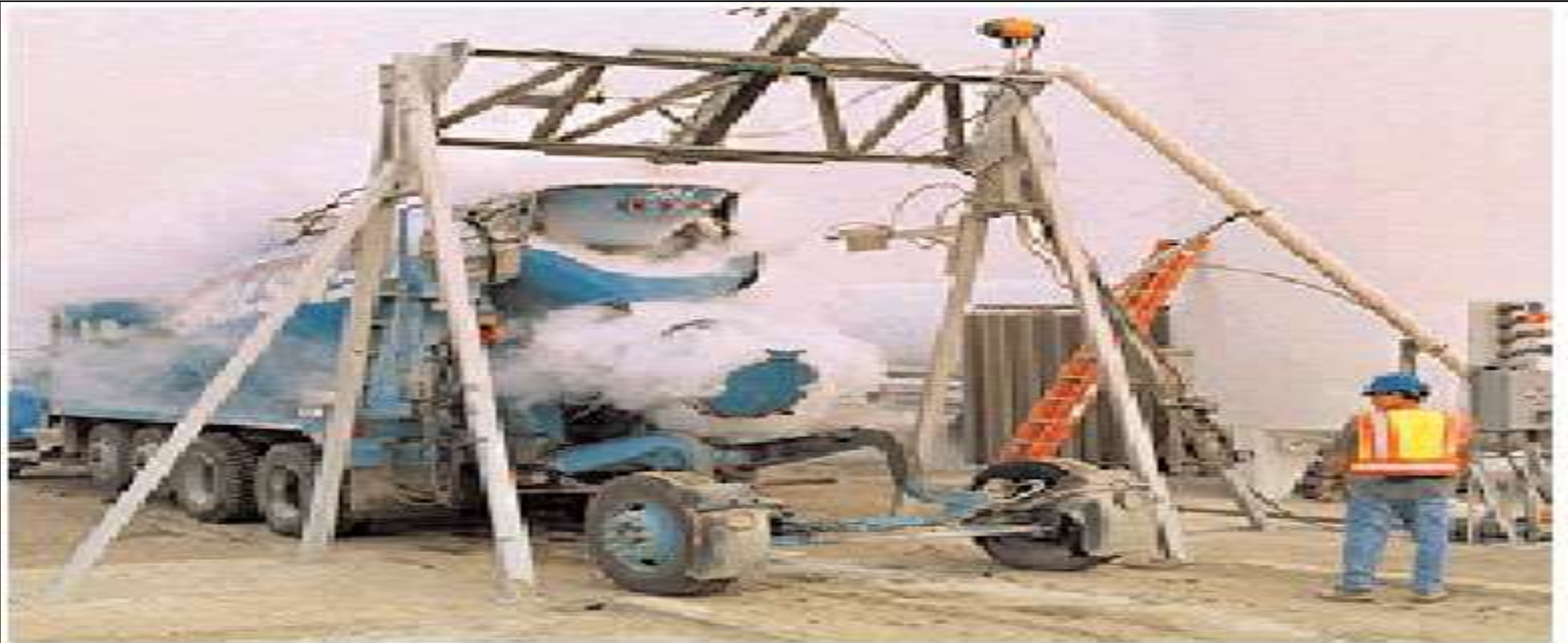
Fig. 13-1. Liquid nitrogen added directly into a truck mixer is an effective method of reducing concrete temperature for delivery to mass concrete placements or during hot-weather concreting. (69954)
