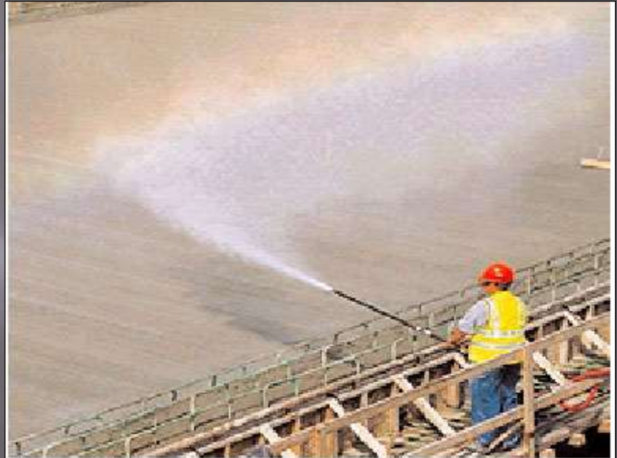
Fig. 13-11. Fogging cools the air and raises the relative humidity above flatwork to lessen rapid evaporation from the concrete surface, thus reducing cracking and improving surface durability. (69956)
