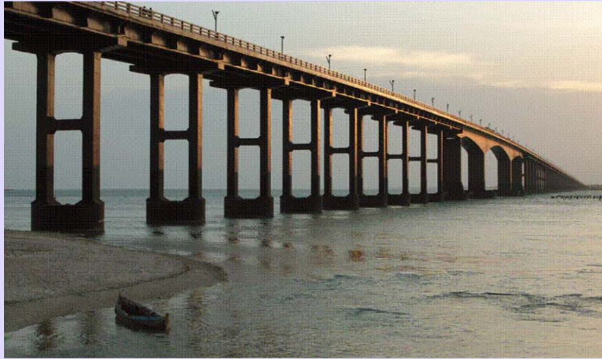
Figure 1-1.8 Pamban Road Bridge at Rameshwaram, Tamilnadu (Reference: http://www.ramnad.tn.nic.in )
